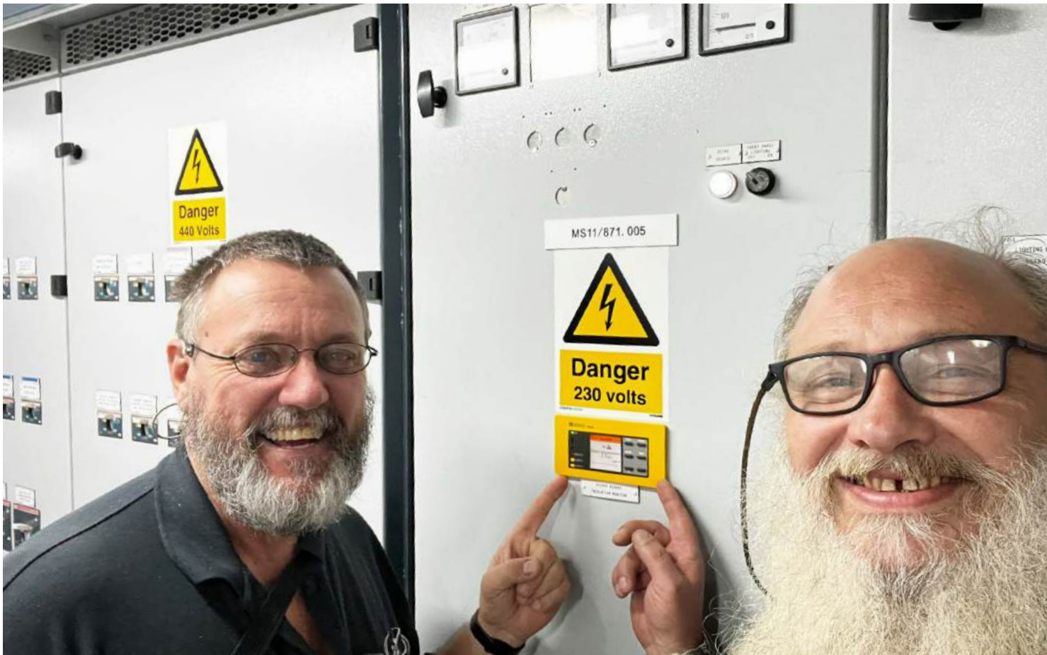
Renier Marx, Chief Electrician, Global Mercy®, Mercy Ships and Alistair Macdonald, Electrical and Control Technician, are delighted about the automatic fault location in the main and emergency switchboard.
