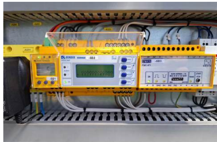
Slim device on the left: LPR measurement (Low Parallel Resistance) Two devices on the right: HPR measurement (High Parallel Resistance)
