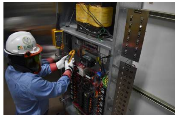
For the re-certification of the systems in accordance with the requirements of applicable standards, faults are simulated, and the triggered alarms are checked.
